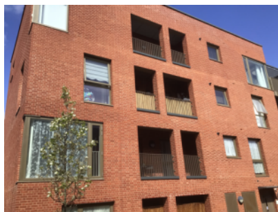
Showing external walls with balconies front elevation
