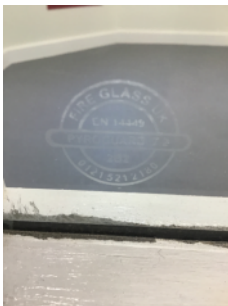
Acid etching, on staircase door glazing
