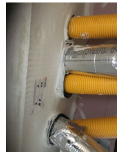
Fire stopping around pipes with intumescent collars fitted
