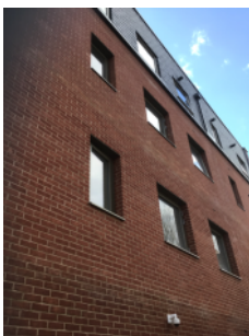
External walls rear elevation
