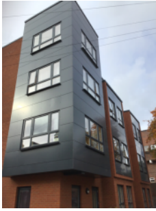
External wall system installed on NE elevation of building
