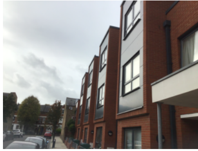
Brick/mortar external walls with an unidentified material window rainscreen
