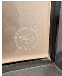
Acid etching of flat door glazing
