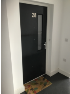
Typical example of the standard of a flat entrance door
