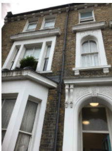
Original brick exterior walls
