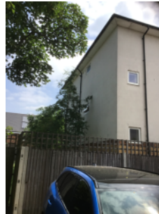
External walls, rear elevation
