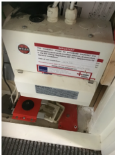
Electrical installations inspected May 2017
