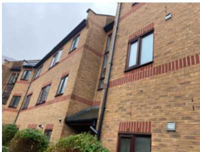
External walls - front elevation
