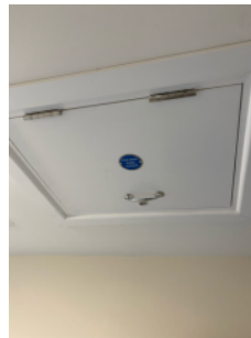
It was not possible within the scope of this FRA to access the roof space
