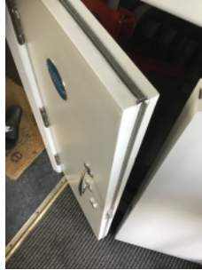
Intumescent strips and cold smoke seals fitted in electrical cupboard doors
