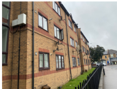
External walls - rear elevation (road side)
