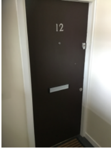
Typical example of flat entrance door in the building
