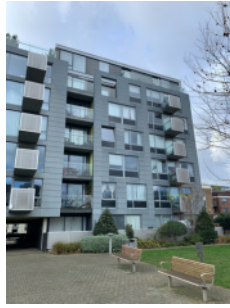
Unidentified cladding system on buildings exterior.
