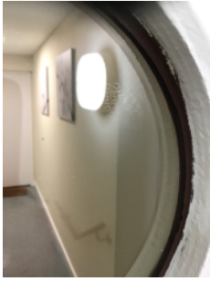
Staircase door glazing, showing "Pyroguard" acid etching
