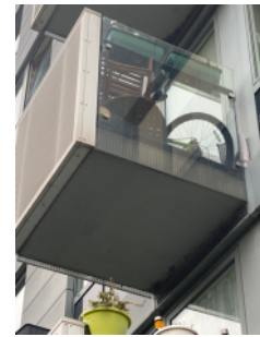
Steel construction private balconies with glazed upstands
