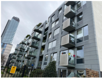
Unidentified (metallic) EWS - rear of building
