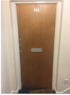
Example of a typical flat entrance door in the building.
