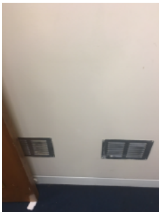
Confirm grill-vents are intumescent protected
