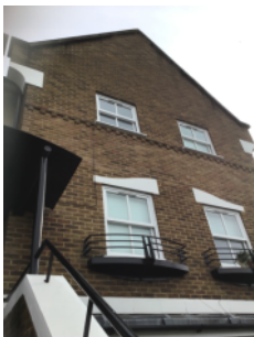
Brick and mortar external walls
