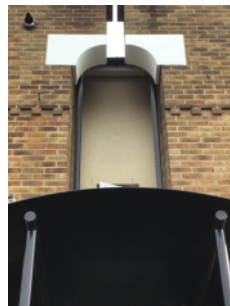
Rendered recess above main entrance door
