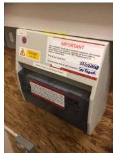
Evidence of testing of fixed electrical installations
