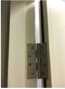
Intumescent strips and cold smoke seals, with CE1121 hinges in riser doors
