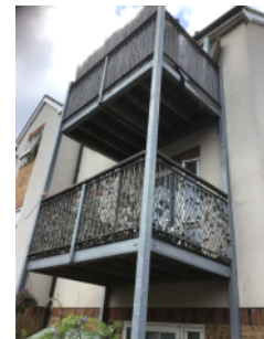
Construction of private balconies
