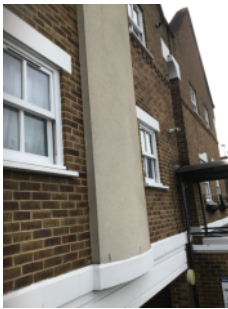
External walls - brick and mortar construction, rendered central column
