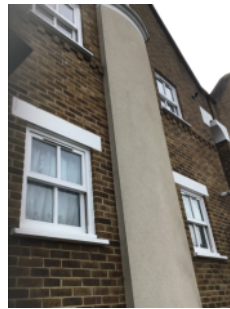
Mortar rendered central column on front face of building
