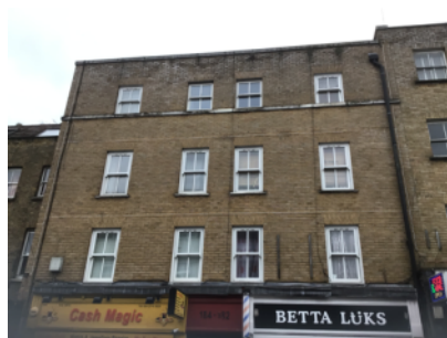
Front elevation – brick/mortar construction
