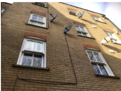
External walls – rear elevation, brick/mortar construction.
