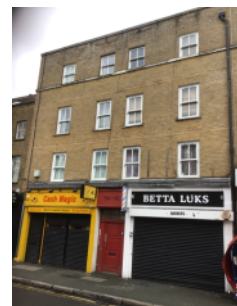
Flats occupying 1st, 2nd and 3rd floors with retail outlets ground floor.
