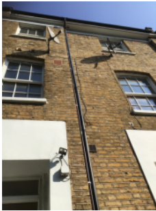
Brick external walls
