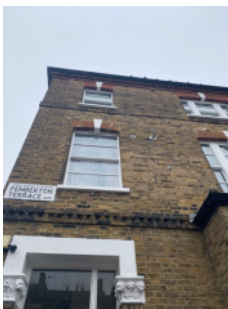
Front elevation - original brick/mortar walls
