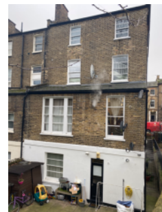
Rear elevation - original brick/mortar walls, with render to lower ground.
