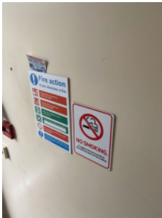
Fire action notice and “no smoking” signage.
