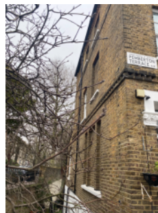
Side elevation - original brick/mortar walls
