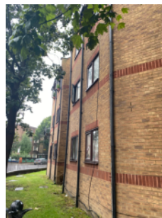
External walls - rear elevation
