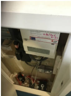
Electrical installations inspected May 2016
