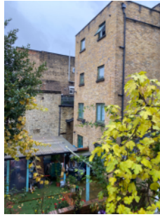
Brick/mortar external walls - rear elevation
