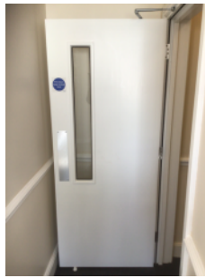
Example of lobby door provided in the building
