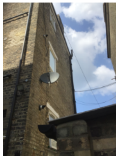
External walls – side elevation.
