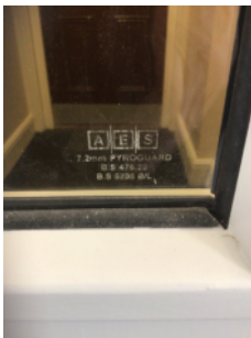
Acid etching on staircase door glazing.
