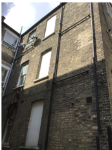
External walls - rear elevation.
