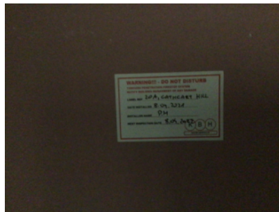
Evidence of fire stopping in lower ground floor electrical cupboard
