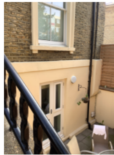
External walls - front elevation
