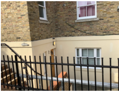
External walls - rear elevation
