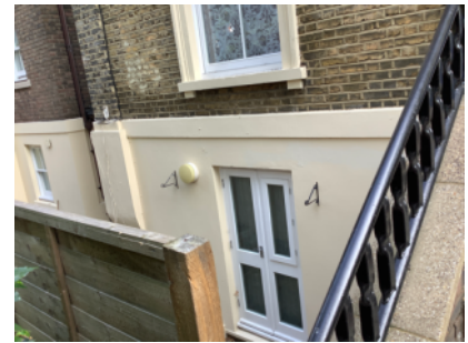
External walls - front elevation
