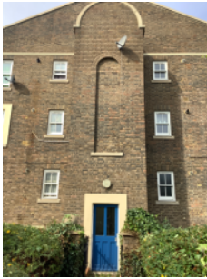
Brick/mortar external walls- rear elevation
