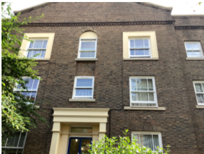
External walls- front elevation
