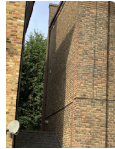
Brick/mortar external walls- end elevation
