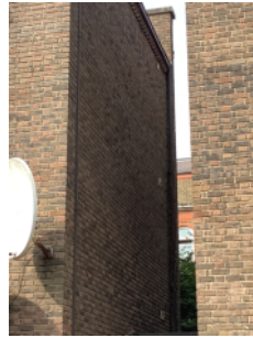
Brick/mortar external walls- end elevation
