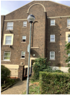
External walls - rear elevation
