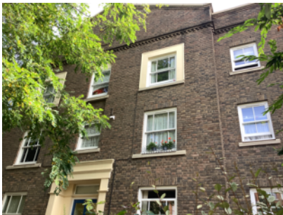
External walls - front elevation
