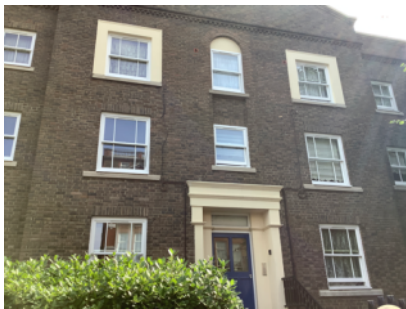
External walls - front elevation
