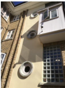
External walls front elevation
