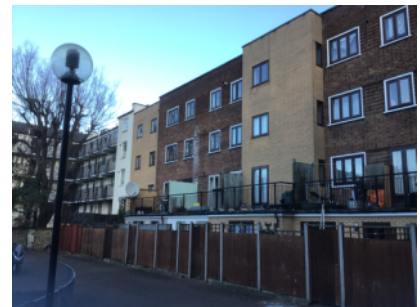
Rear elevation- brick/mortar walls, private balcony on 1st floor.
