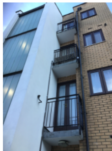
Brick/mortar external walls, with rendered section around the staircase
