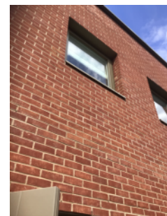
External walls rear elevation
