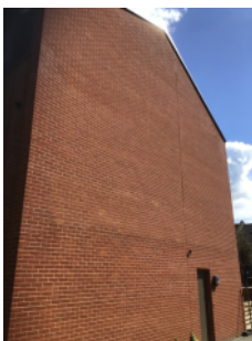
Brick and mortar construction end elevation
