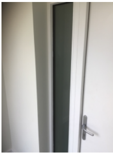
Glazed panels on flat entrance doors.
