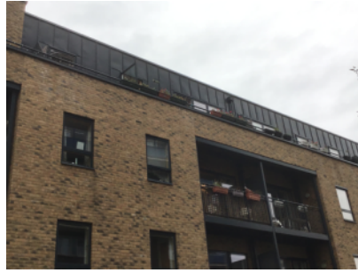
Metallic cladded external wall system on fourth (uppermost) floor.
