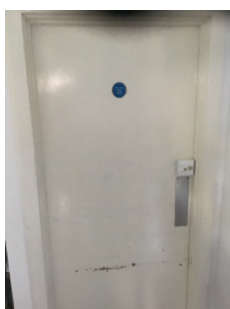
It was not possible to access this door due to availability of a key.
