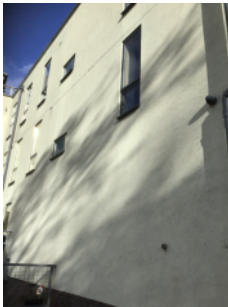
External walls - rear elevation
