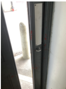
Thumb turn on main entrance door
