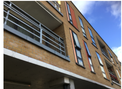
External walls - front elevation
