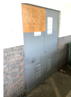
It was not possible to access this room due to key availability
