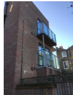
Private balconies- rear elevation
