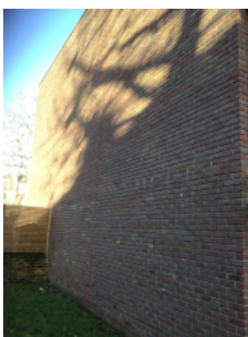
Brick/mortar external walls- side elevation
