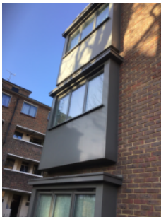
Metallic rainscreen/cladding section around windows at the front elevation
