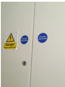
Electrical cupboard doors.
