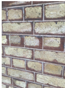
Original brick/mortar external walls
