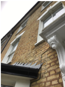
Original brick/mortar external walls
