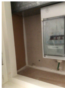
Construction within electrical cupboard
