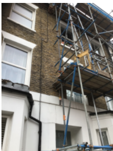
Brick and render front facade of the building
