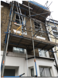
Scaffold erected on front face of the building
