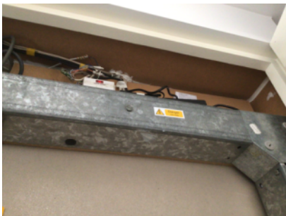
Construction within the electrical cupboard
