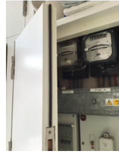
FD30S construction enclosing electrical installation
