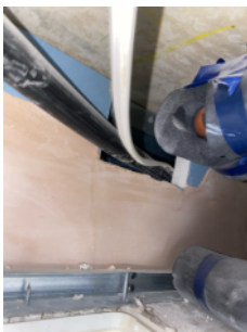
Cable penetrations into the smoke shaft, above ceiling outside flat 22
