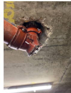
Pipe penetration through a concrete slab within the bin store.
