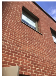
External walls rear elevation
