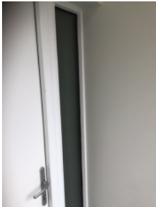
Glazed panels on flat entrance doors.
