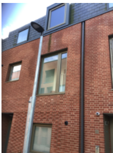
Brick/mortar construction, with tiled facade on second floor
