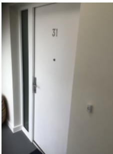
Example of flat entrance door.
