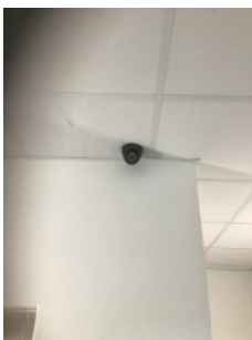
CCTV provided internally and externally
