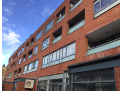
Brick/mortar construction with glazed panels front elevation
