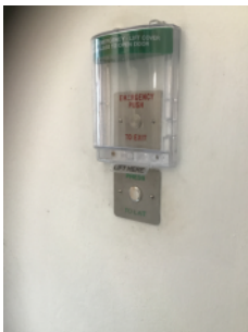
Electromagnetic door release with emergency release device
