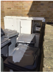
External bin store
