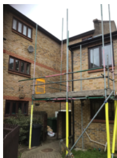
Construction of external walls
