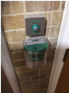
Electromagnetic door release with emergency override
