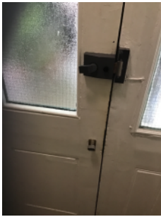
Thumb-turn device on main entrance door
