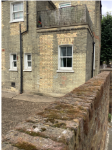
External walls - rear elevation
