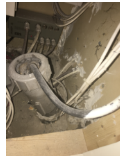
Some fire stopping has been installed in the electrical cupboard
