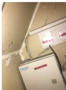
Some fire stopping has been installed in the electrical cupboard
