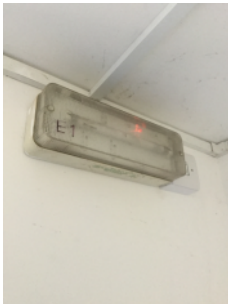
Non-maintained emergency light unit
