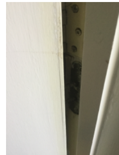
Concealed door jamb closer on entrance door to Flat A.
