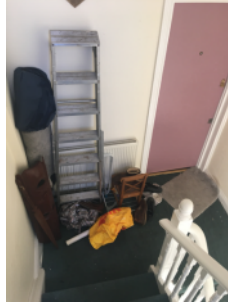
Combustibles in the common area.
