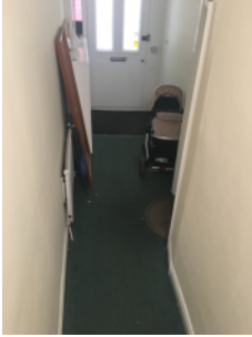
Combustibles in the common area.
