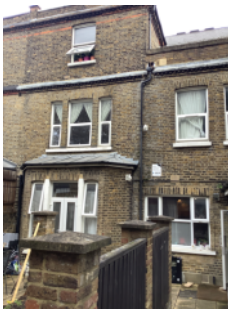
External walls - rear elevation
