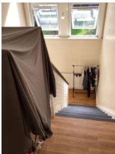
Drying racks in escape route
