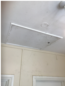
It was not possible to access the loft space
