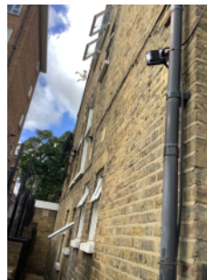
External walls side elevation
