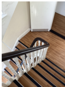
Escape route with contrasting stair nosings
