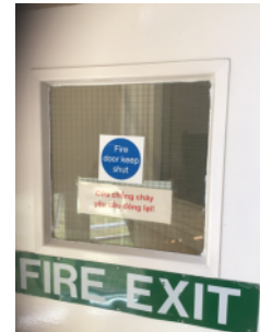
Georgian wired glazing installed in lobby doors
