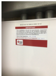
Evidence of fixed electrical installation testing in May 2019
