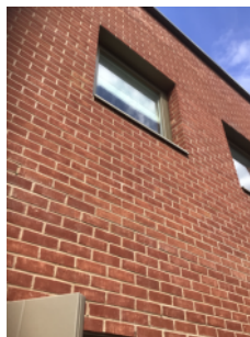
External walls rear elevation
