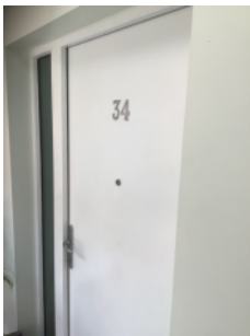
Example of flat entrance door.
