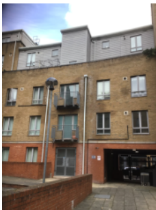
External walls - rear elevation
