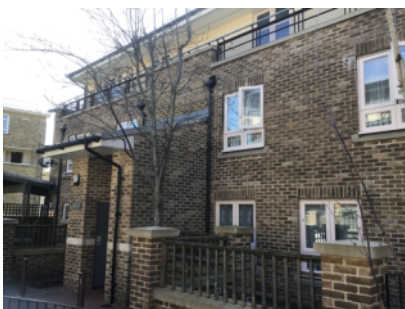
External walls front elevation.
