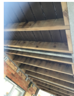
Timber balcony deck construction
