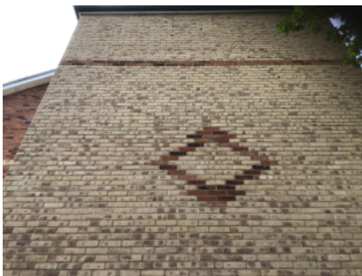
Brick/mortar external walls- side elevation
