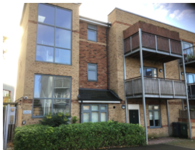
Brick/mortar external walls- front elevation
