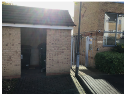
Bin store located externally and away from main building
