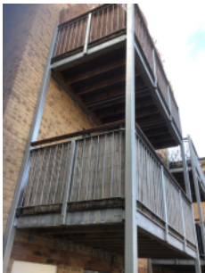
Steel framed balconies with timber deck
