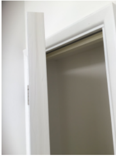
FD30S riser door with intumescent strips and smoke seals fitted into frame
