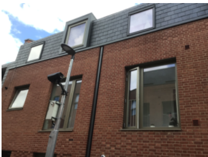
Brick/mortar construction, with tiled facade on second floor
