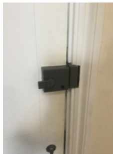
Latch on main entrance/egress door.
