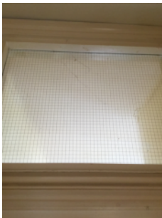
Georgian wired fanlight above lounge door in Flat D
