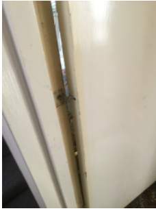
Concealed door jamb closer to entrance door of Flat D
