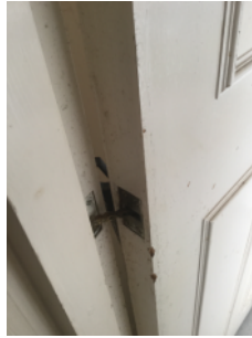
Concealed door jamb closer on lounge door.
