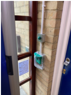
Electromagnetic door release and emergency door release
