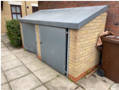
Bin store located away from the building.
