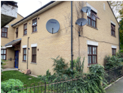
Brick/mortar external walls- front and side elevation
