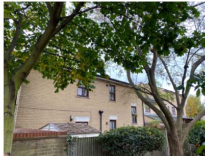
Brick/mortar external walls - rear elevation
