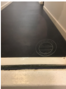
Acid etching on door glazing
