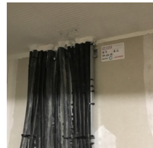
Evidence of fire stopping
