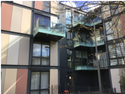
External walls and balconies, rear elevation
