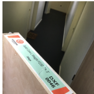
New riser cupboard doors
