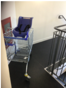
Obstructions in staircase
