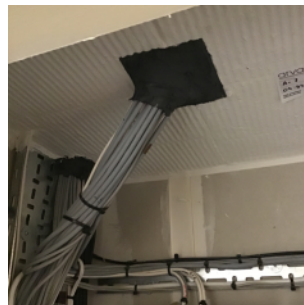
Evidence of fire stopping
