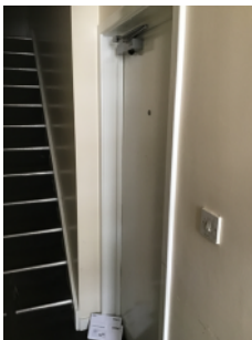
Example of typical flat entrance door (flat A)
