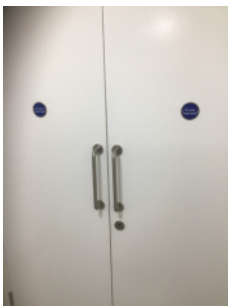
“Fire door keep locked” signage on the riser cupboard doors
