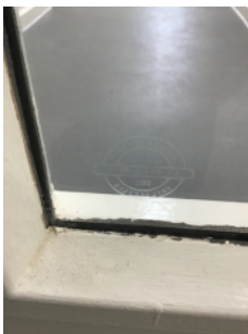
Acid etching, on staircase door glazing
