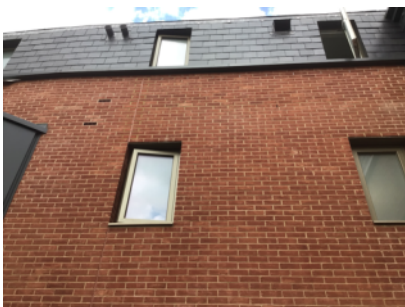
External walls – rear elevation.
