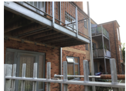
External walls -end elevation
