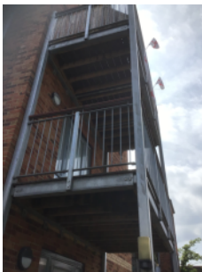
Construction of private balconies
