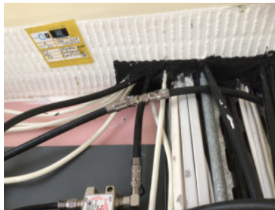
Fire stopping within riser cupboards.
