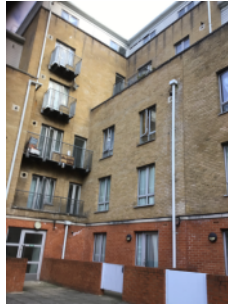
External walls-rear elevation.
