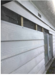
External wall system fixed to timber battens on fifth floor.
