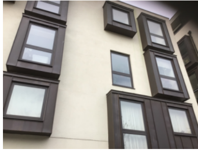
External walls - front elevation
