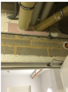
Fire stopping in basement
