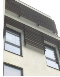
Decorative gridwork (timber) attached to 3rd and 4th floor external walls
