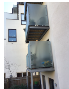
Timber decked balconies
