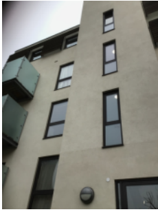
External walls – rear elevation.
