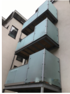
Construction of private balconies on rear elevation of the building
