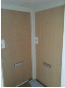
All flat entrance doors of the same appearance.
