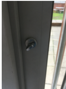
Thumb turn device on rear exit door.
