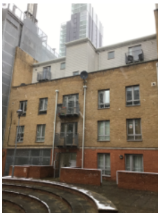
External walls - rear elevation.
