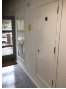
New fire resisting doors have been fitted to all riser cupb
